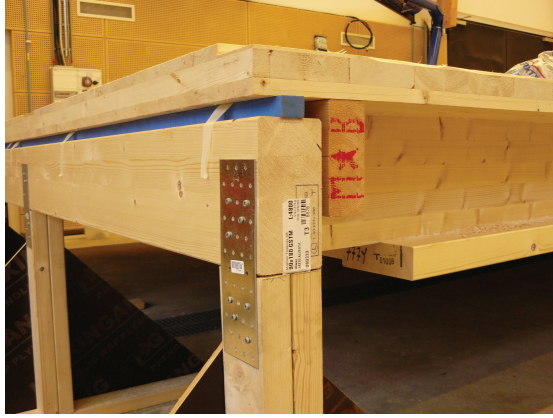
Figure 10: Floor supports joined to a glulam beam by means of a tie plate, the floor resting on top. In this case, the floor is required to rest on top of an elastomer, blue in colour in the picture, according to the manufacturer's instructions.
