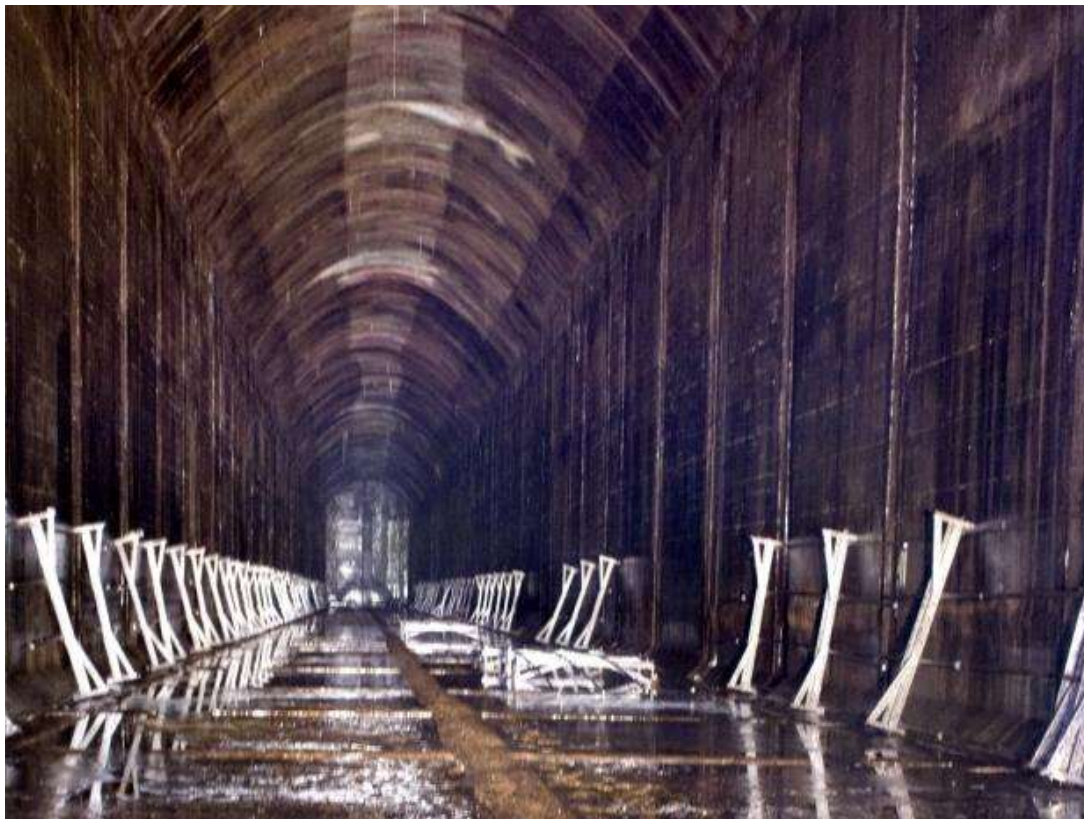
The oil-storage complex at Inchindown, near Invergordon in Scotland, was built during the Second World War
